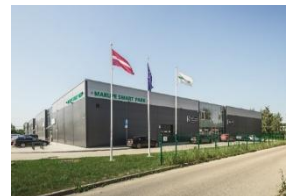
Industrial MARUPE Riga, Latvia GLA: 6 182 m 2 Occupancy: 68 %
